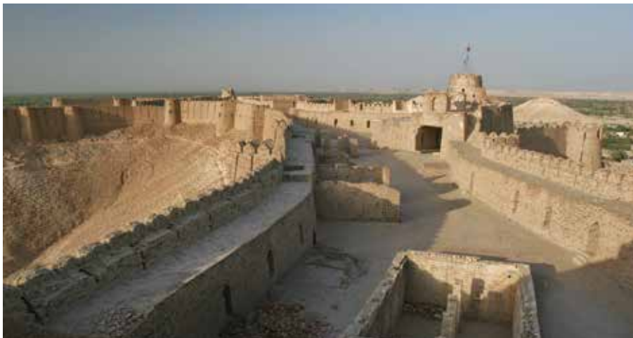
Figure 4: The defensive wall of Kot Diji Fort Sindh, Pakistan.
